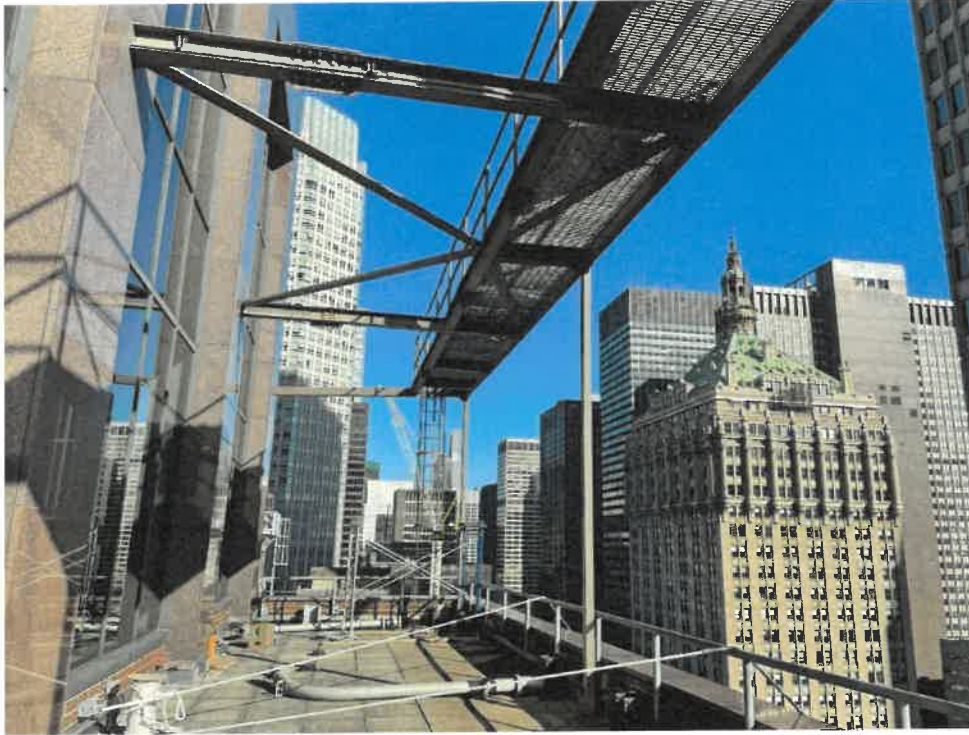
Photo 7: - Framing of North Structure.
