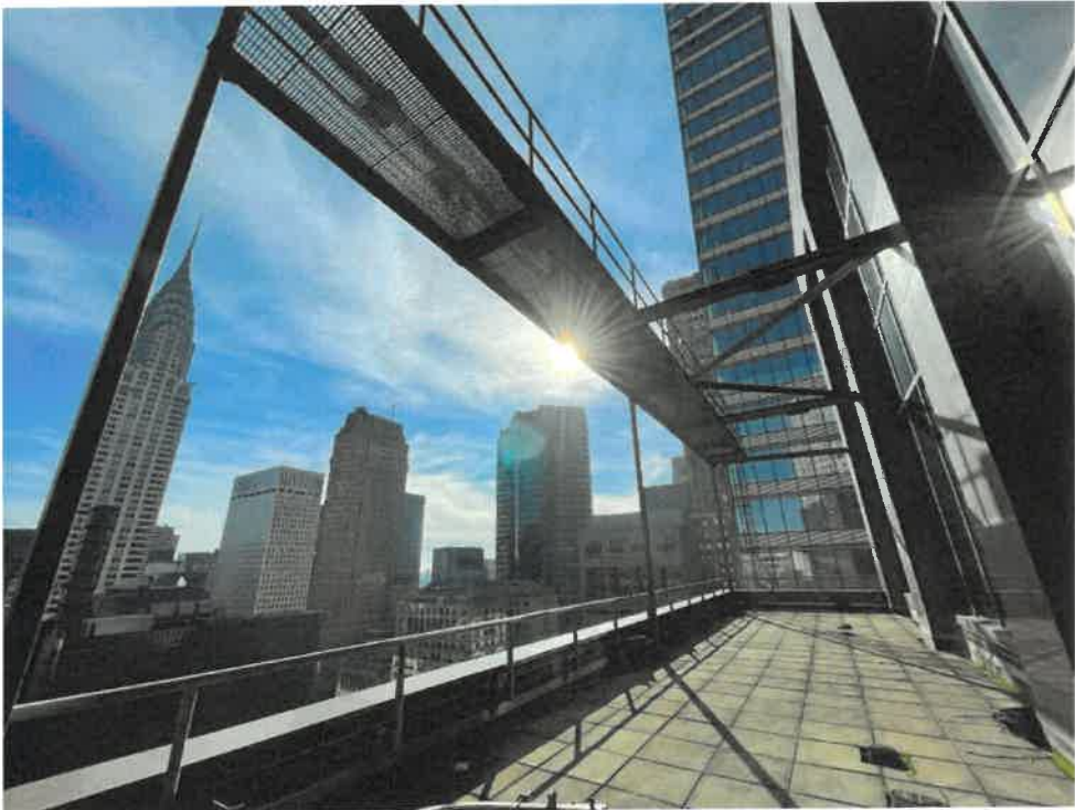
Photo 11: - Framing of South structure.
